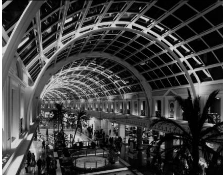
Figure 2.3 Curved roof steelwork to retail centre
