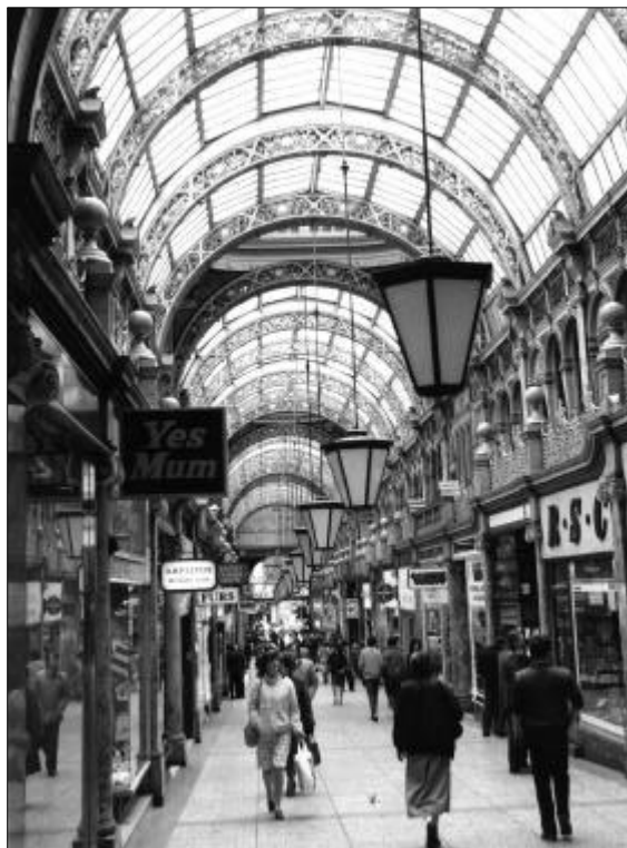
Figure 2.1 Curved cast iron roof trusses
