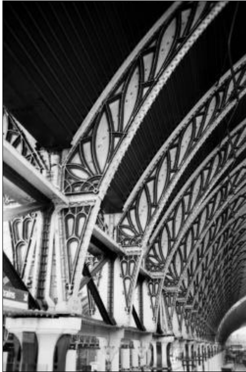
Figure 2.2 Curved wrought iron with decorative cast iron inserts
