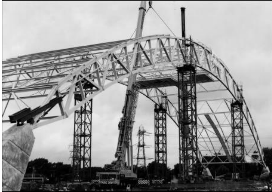
Figure 2.5 Curved trusses for sports facility
