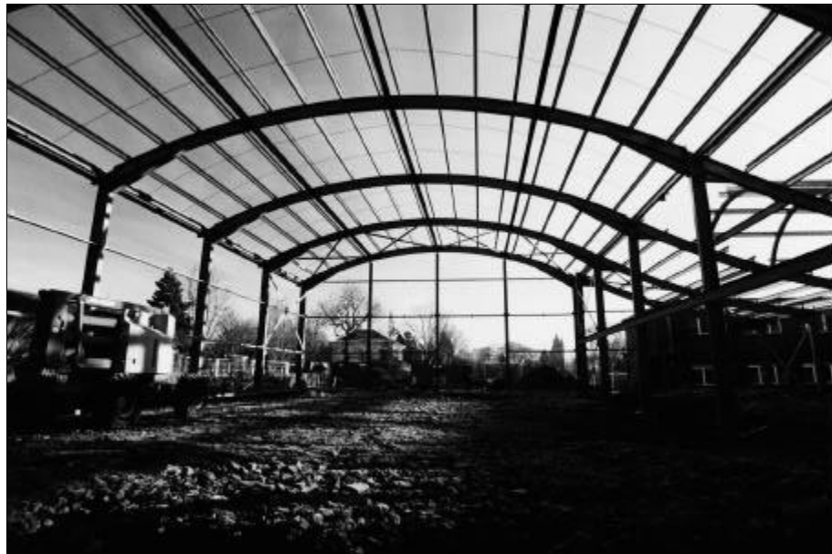
Figure 2.4 Portal with curved rafters
