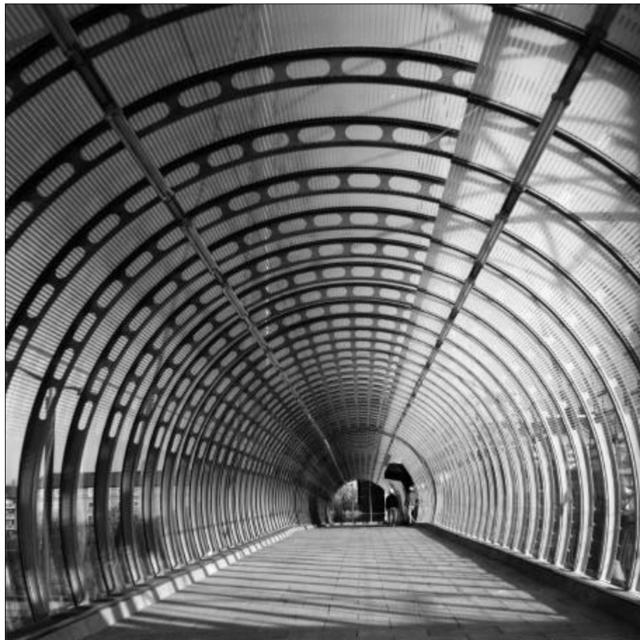
Figure 2.6 Curved steel supports for walkway enclosure
